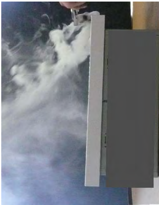
FIG. 1 BRAND K SMOKE TEST
